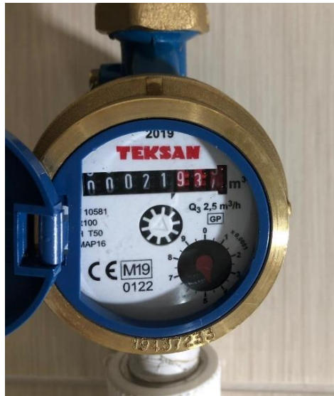
Figure 3.1 Used flowmeter in the toilet
