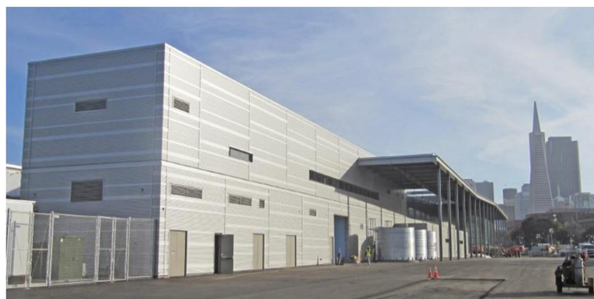
Figure 2.13 Three aboveground rainwater collection tanks at Pier 27
