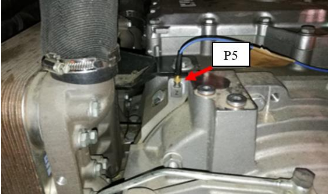
Figure 6.17: Accelerometer instrumentation for P 5
