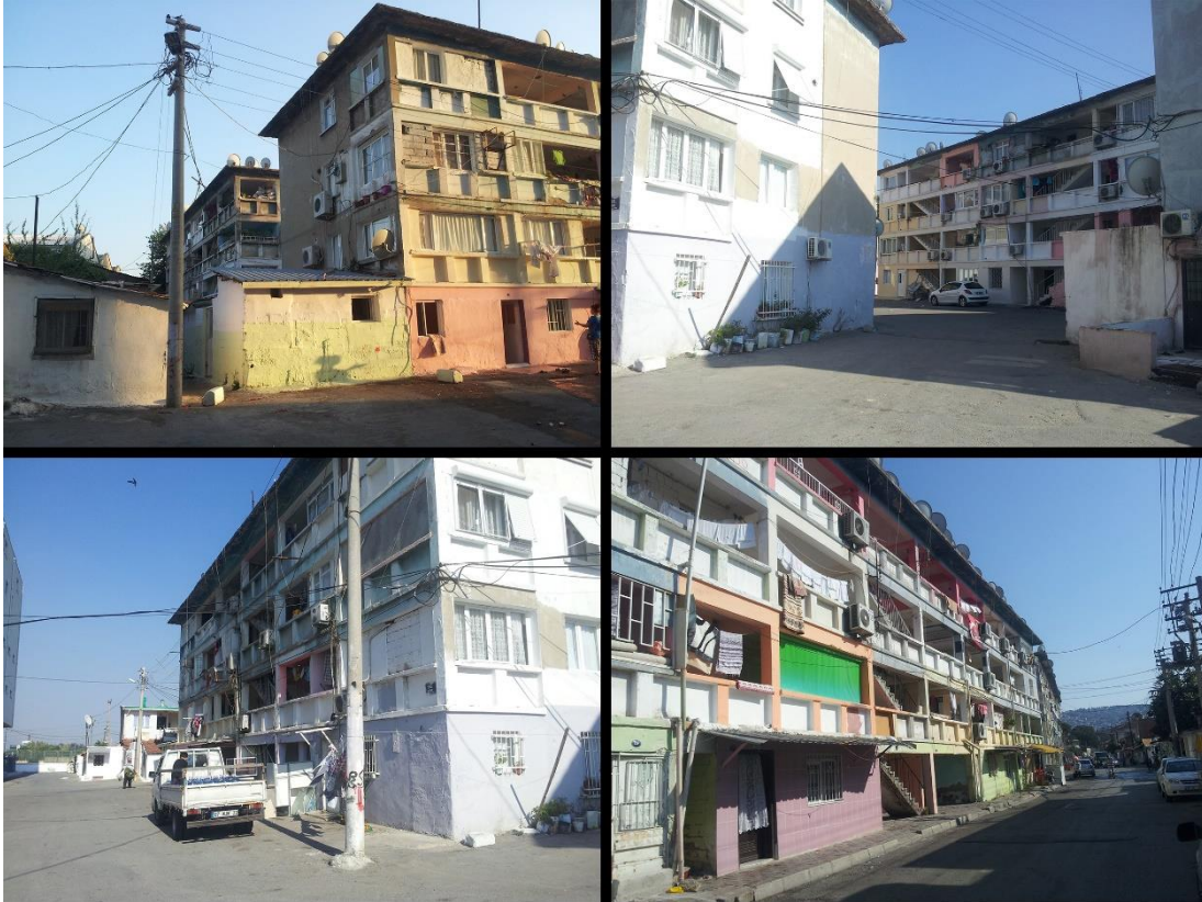
Figure 5.11: Apartment blocks in Ege neighborhood
