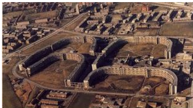
Figure 2.4. Hulme`s crescent blocks of 60s regeneration project.
