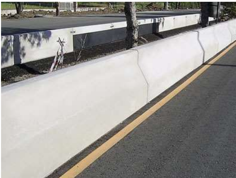
Figure 1.2 : Concrete Barrier (URL 2).
