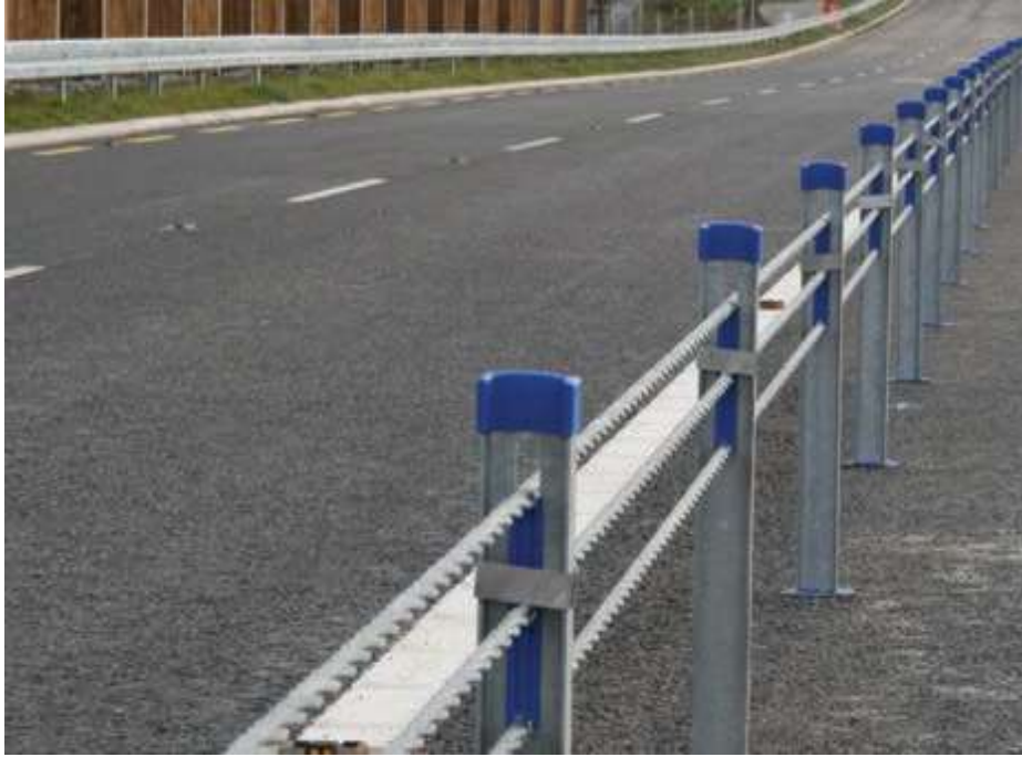
Figure 1.3 : Wire Rope Barrier (Yeginobali, Atahan et al.).
