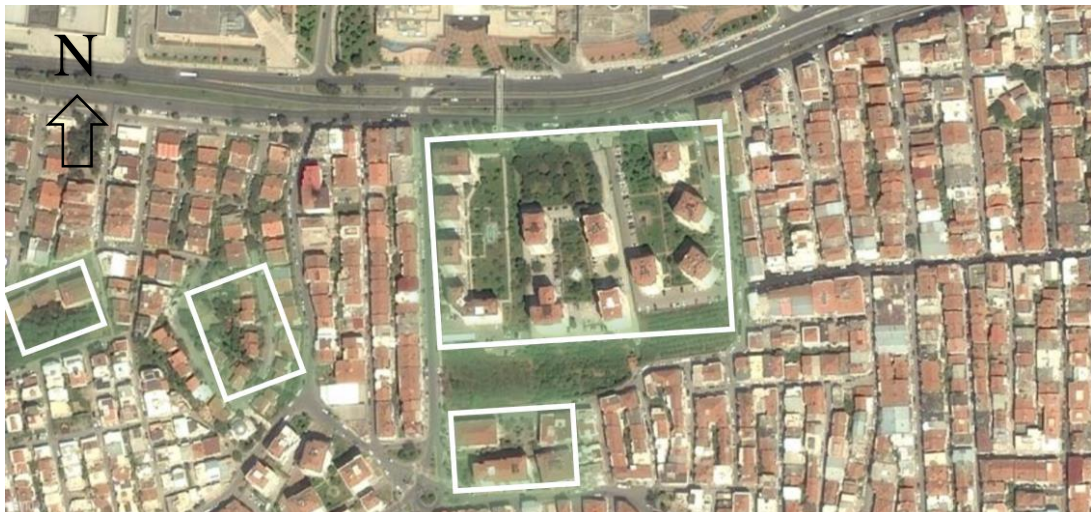
Figure 5.8 : Settlement from Narlıdere district
