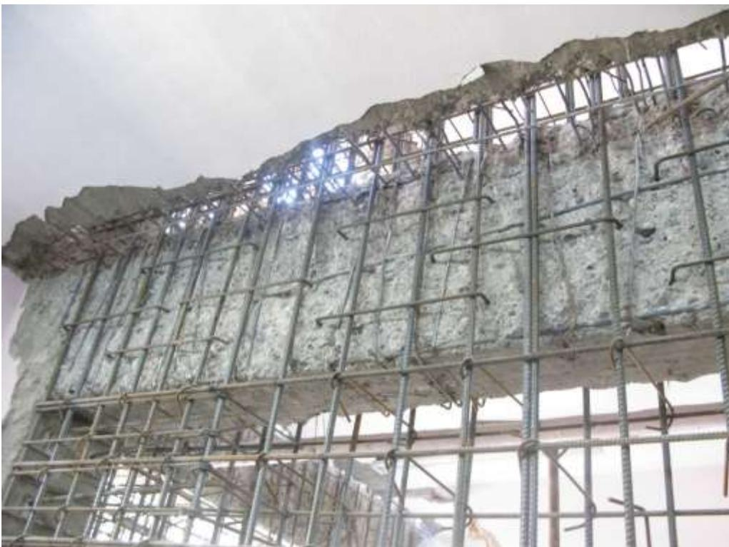
**Figure 1.3 :** Anchors functioning as cross-ties.
