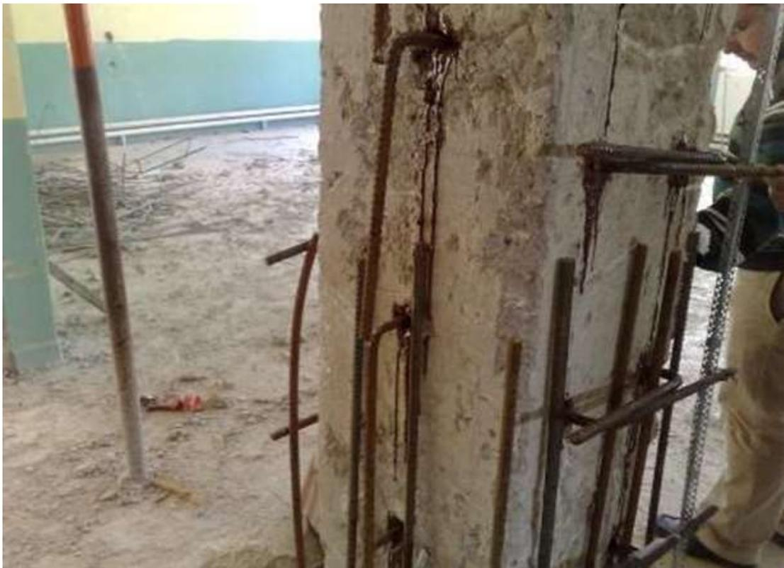
**Figure 1.1** : Anchors in jacketing of column [4].
