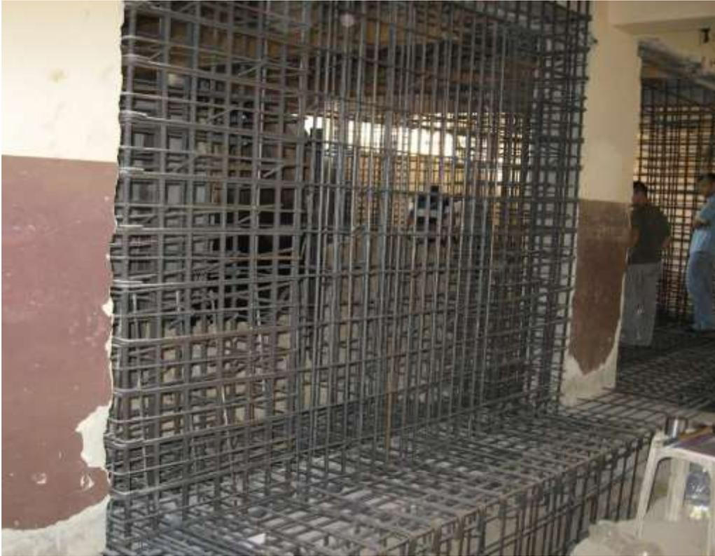
**Figure 1.2 :** Anchors connecting infill shear wall to frame.
