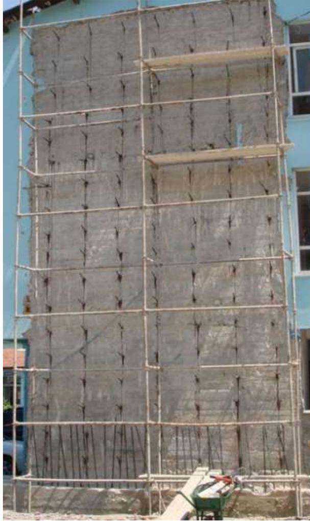
**Figure 1.4 :** Anchors in external shear wall application [4].
