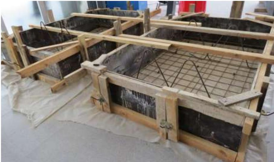
**Figure 3.6 :** Mold prepared for pouring of concrete
