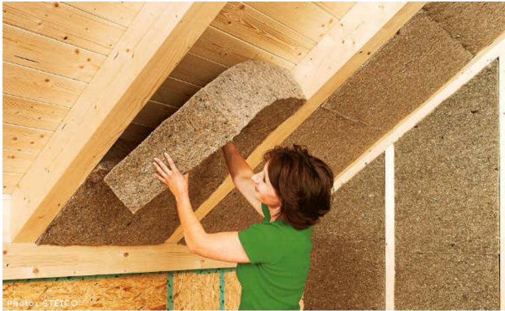
Figure 3.17 : Roof being insulated with hemp panels.
