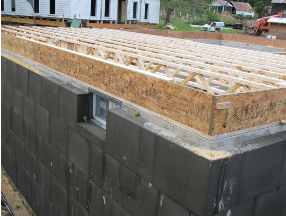
Figure 3.8 : Basement floor walls insulated with foam glass.
