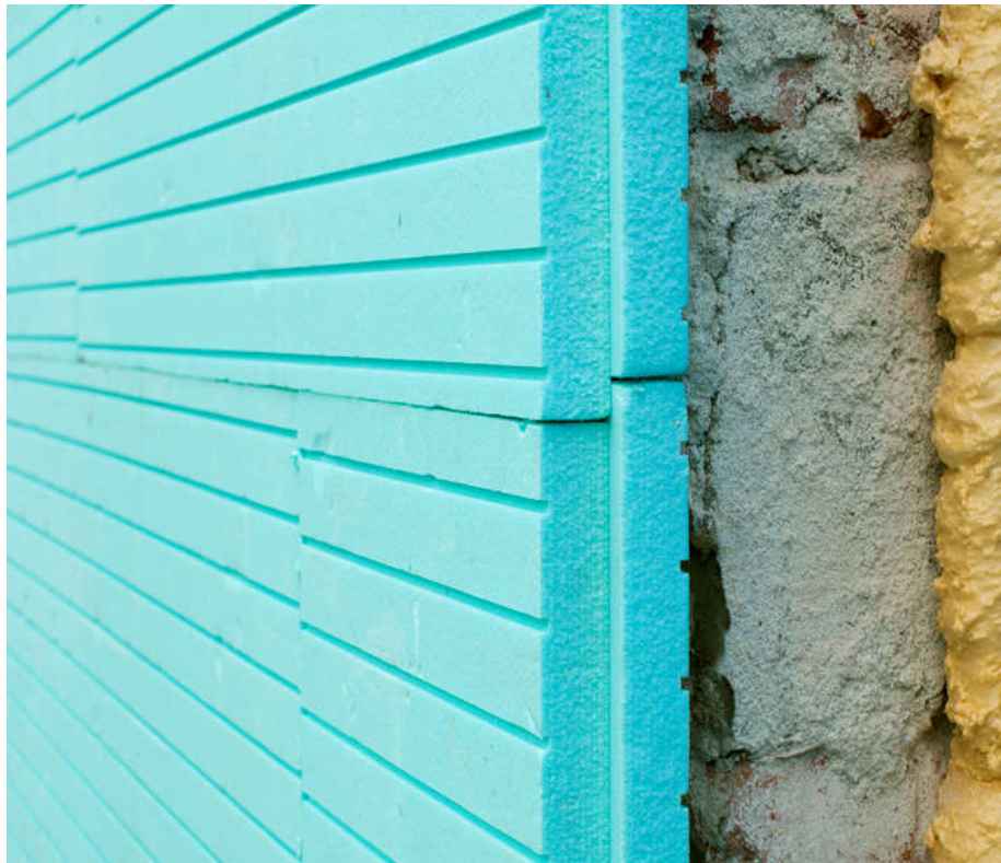
Figure 3.12 : Wall being insulated with XPS panels.
