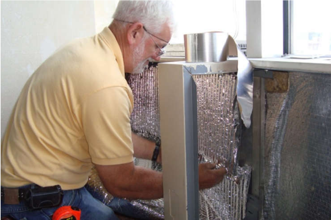
Figure 3.39 : GFP being applied for insulation.
