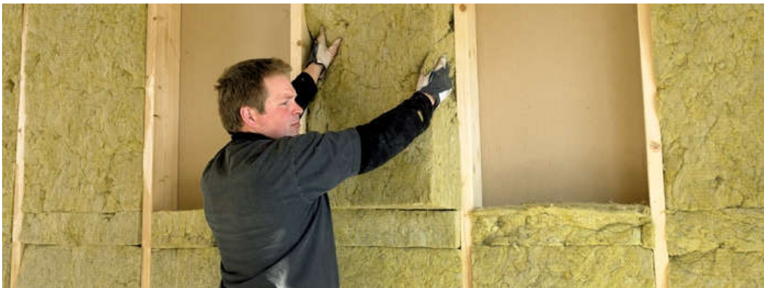
Figure 3.6 : Wall insulated with rockwool.
