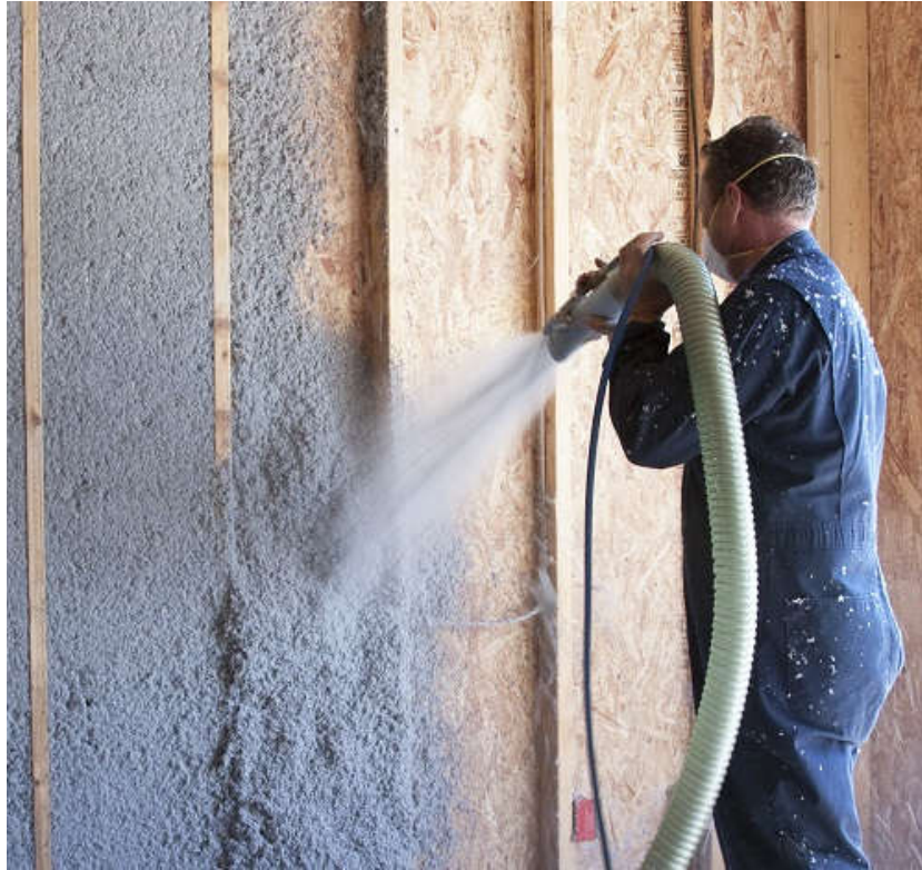
Figure 3.44 : A wall being insulated with cellulose.
