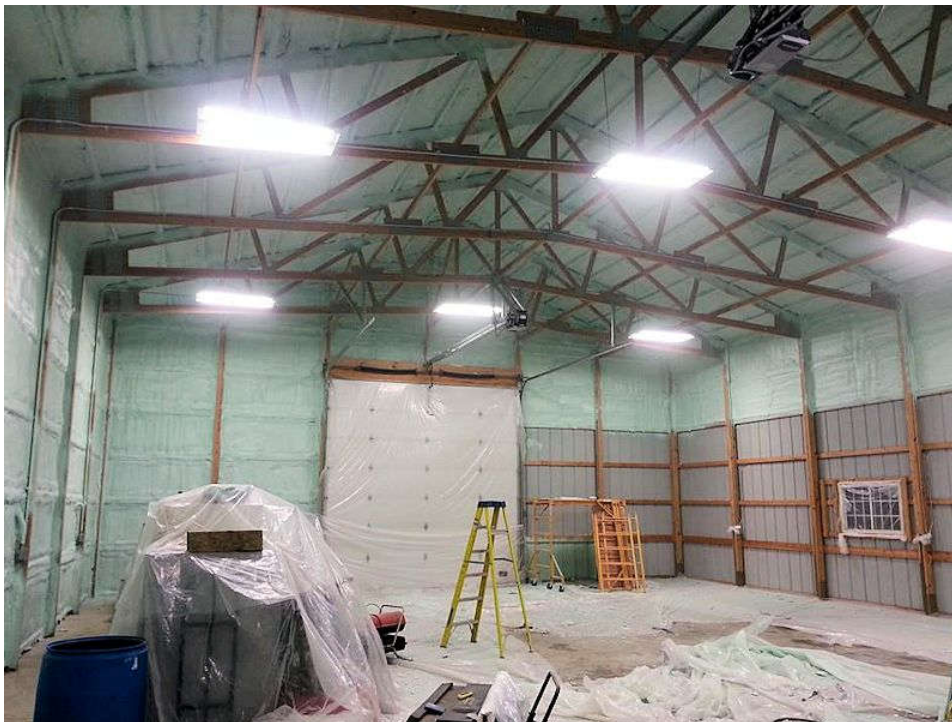
Figure 3.19 : Industrial construction being insulated with soy based insulation.
