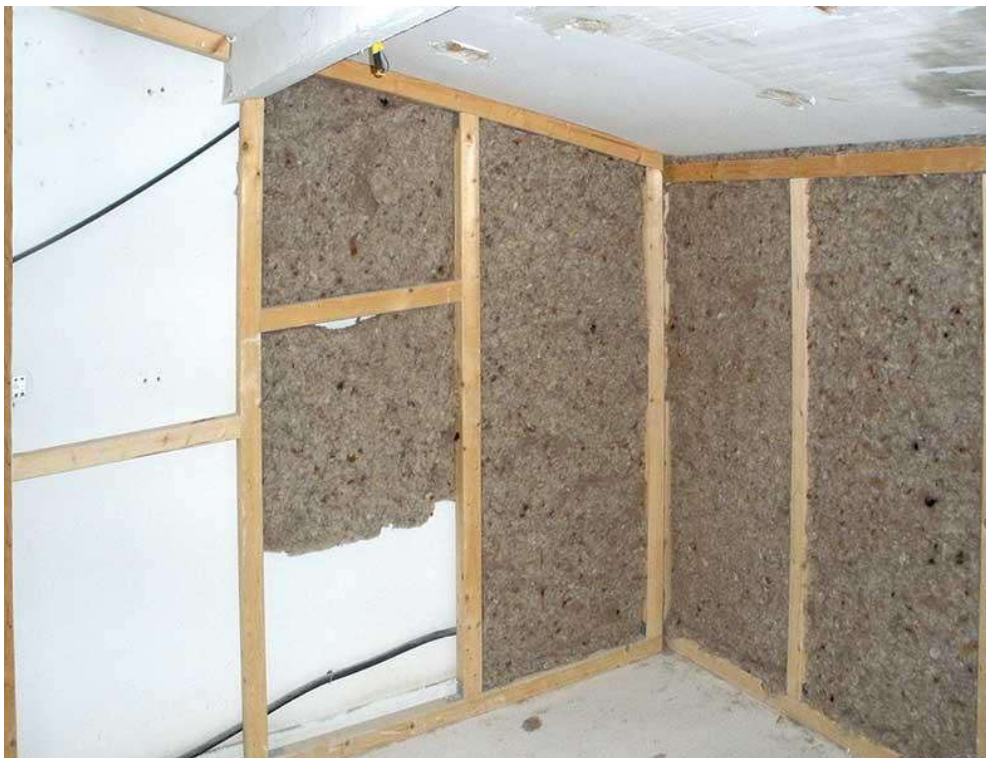
Figure 3.23 : A wall being insulated with sheep's wool insulation.
