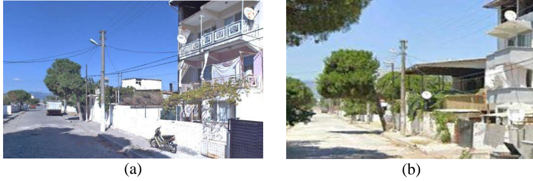
Figure 4.3: Photos of building number 70, (a) From 2016, (b) From 2022.
