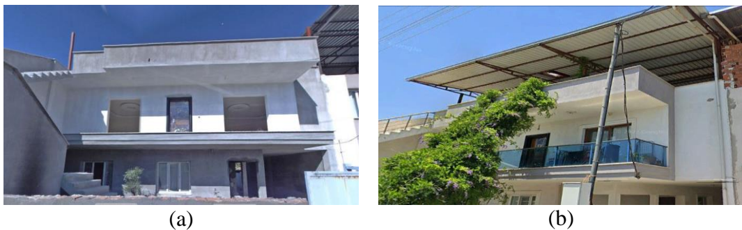
Figure 4.2: Photos of building number 65, (a) From 2016, (b) From 2022.
