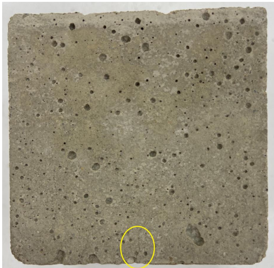
Figure 4.143: Freeze-thaw cracking on the surface of 125ES02 mortar
