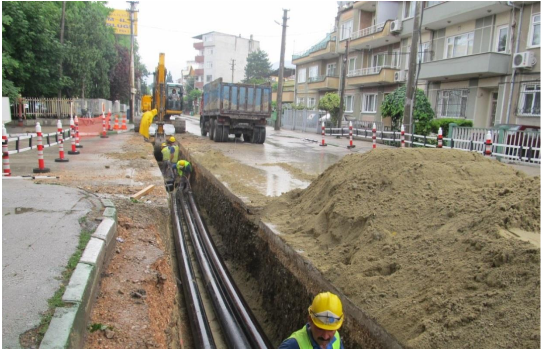
Figure 3.4 : Underground power cable laying process.
