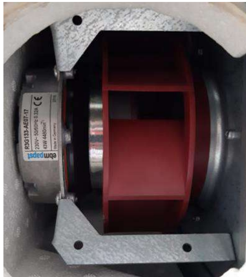
Figure 6. Radials fans in HVAC
