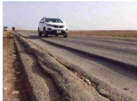
Figure 1. Rutting in Iraq
