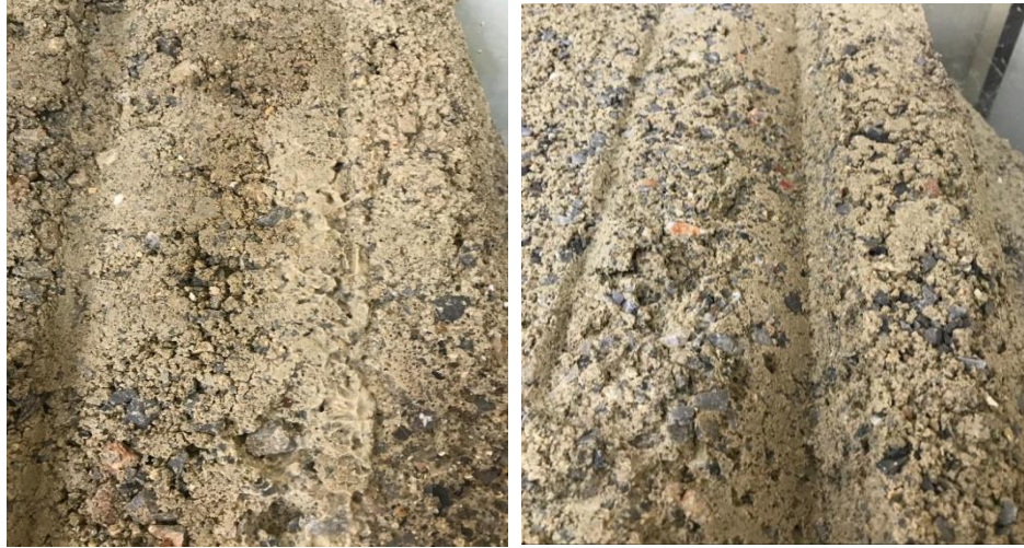
Figure 3. a) Punching of the slope crest, b) Local failure of slope
