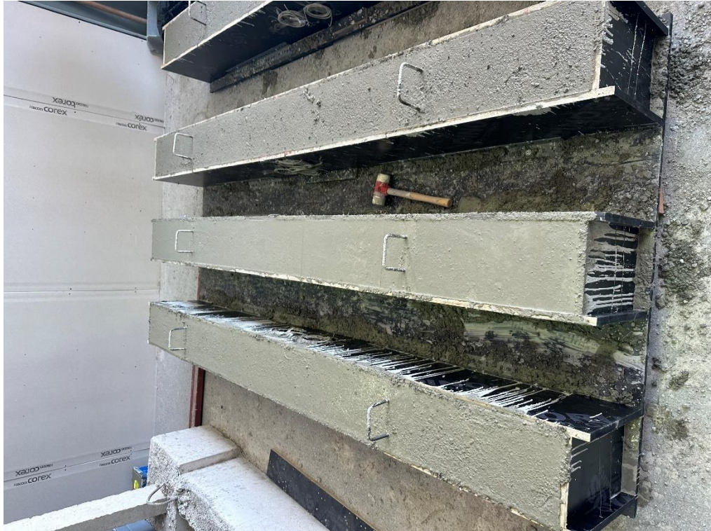
Figure C.3 The beams after concrete pouring
