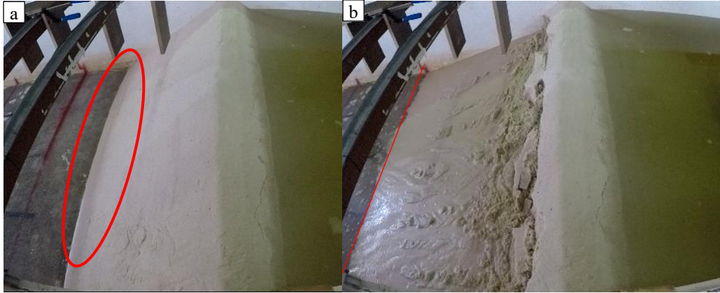
Figure 4.36: Water seepage start from dam body skirt (a) and sediment passing from the red line (b)
